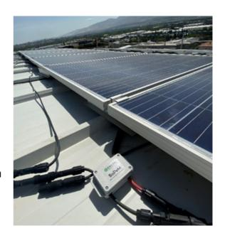
String monitoring system is performed with traditional methods. In case of a malfunction in any panel, the defective panel cannot be determined. SoPeM does panel-based monitoring. In other words, it specifically detects the failure of each panel. It can show the instant value of each panel.
